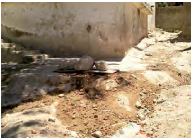
Figure 1: Poorly covered cesspit, June 2012, Photo: FoEME
