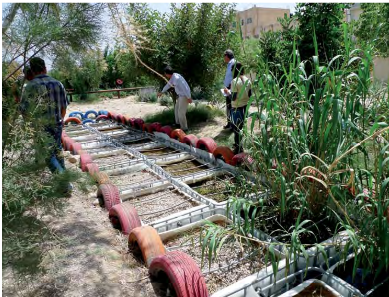
Figure 3: Ecological greywater treatment system at Auja Eco-Center, Photo: FoEME
